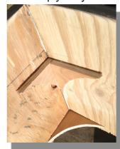
offcuts from front and back used as locating blocks for roof saving material
